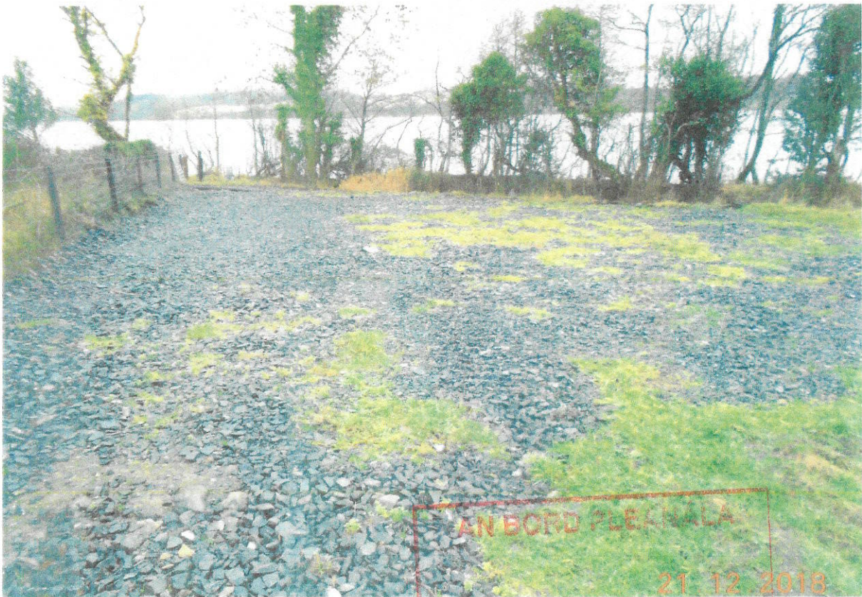
Photo 11 looking northwest from point D on Map 1 showing new turnaround road present within SAC on 21 st of December 2018.
