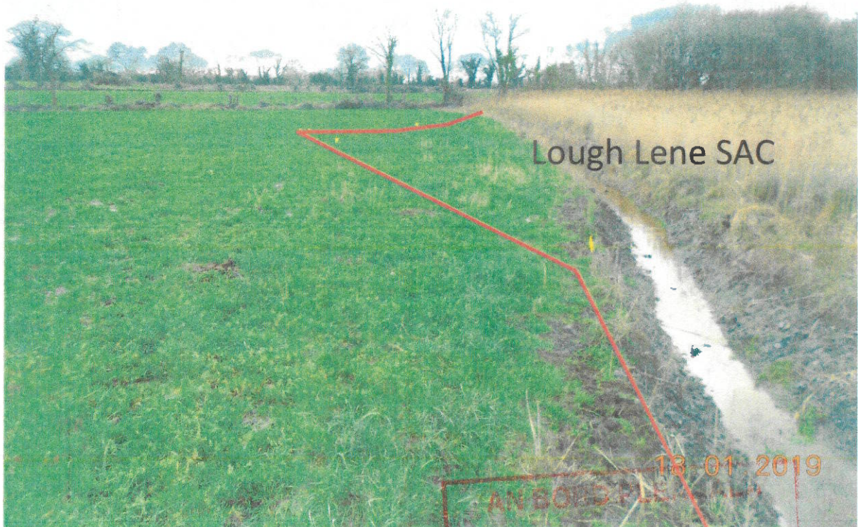
Photo 4 showing one of the areas, west side on Map 3 measuring approximately 0.01ha, of SAC wetland affected by infilling and drainage (right of red line). New drain on right side of photo.
